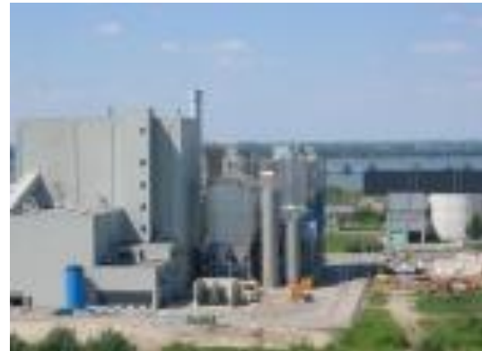
Illustration BMC Moerdijk power plant (The Netherlands). The plant is designed to turn more than 400,000 tonnes/year of poultry litter into electricity (36 MW) and reusable minerals for agriculture. ( http://www.bmcmoerdijk.nl/index.php )
