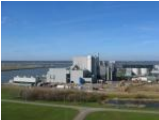
Illustration BMC Moerdijk power plant (The Netherlands). The plant is designed to turn more than 400,000 tonnes/year of poultry litter into electricity (36 MW) and reusable minerals for agriculture. ( http://www.bmcmoerdijk.nl/index.php )
