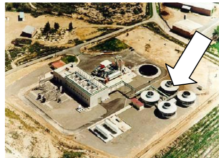
Atmospheric evaporators at the centralized pig manure treatment plants of Alcarras (left) and Altorricon (right), in Spain (GUASCOR technology)
