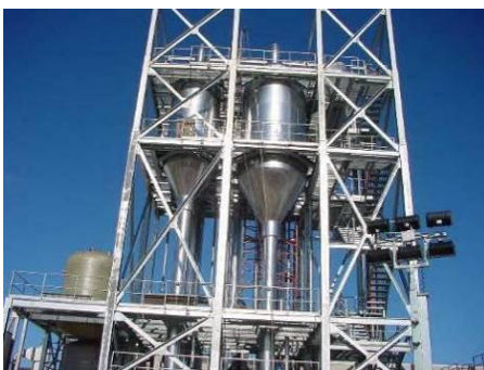
Details of the vacuum evaporation unit at Tracjusa pig manure treatment plant (Juneda, Spain)
