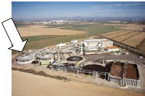
Atmospheric evaporators at the centralized pig manure treatment plants of Alcarras (left) and Altorricon (right), in Spain (GUASCOR technology)
