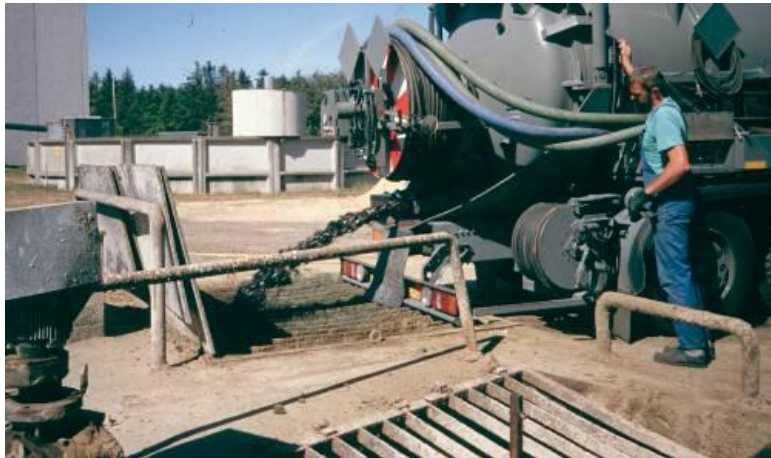
Illustration of separation by grid at the influent of Sending centralized biogas plant (Denmark).
