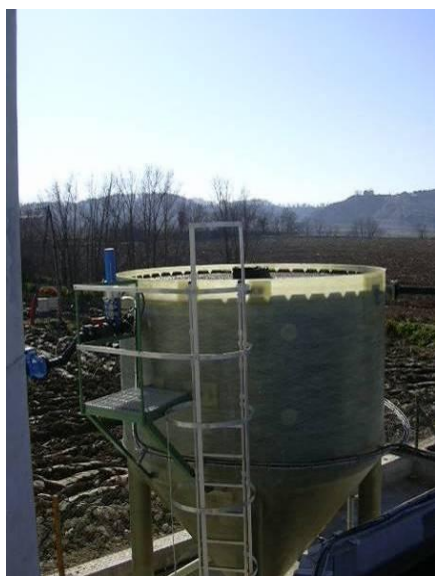
Illustration of a thickener at the pig slurry NDN plant of Calldetenes (Spain)
