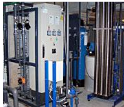
Schematics of the reverse osmosis process (left) and illustration of a cleaning unit with reverse osmosis ( www.kruger.dk )
