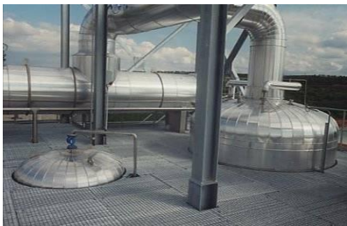
Details of the vacuum evaporation unit at Tracjusa pig manure treatment plant (Juneda, Spain)
